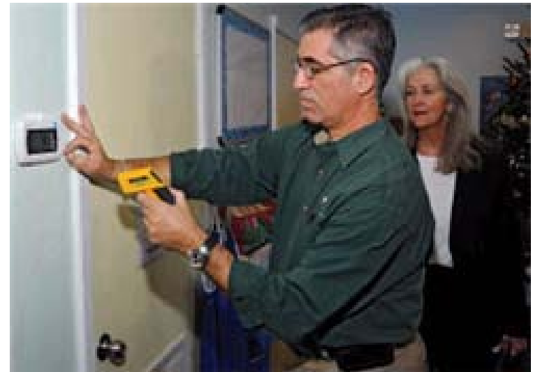
FPL energy expert checks new programmable thermostat installed at Central Brevard Sharing Center as agency board member looks on
